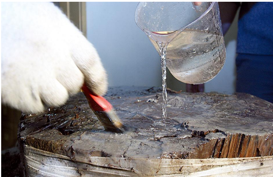
Rinsing the end surface which turned down in the clay
